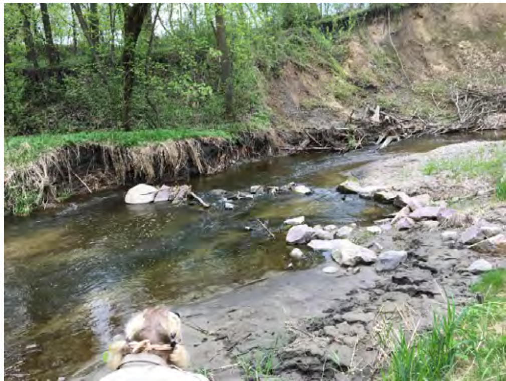
Photo 6-17 Failed vane structure causing bank erosion on left side of photo. 5/14/18.
