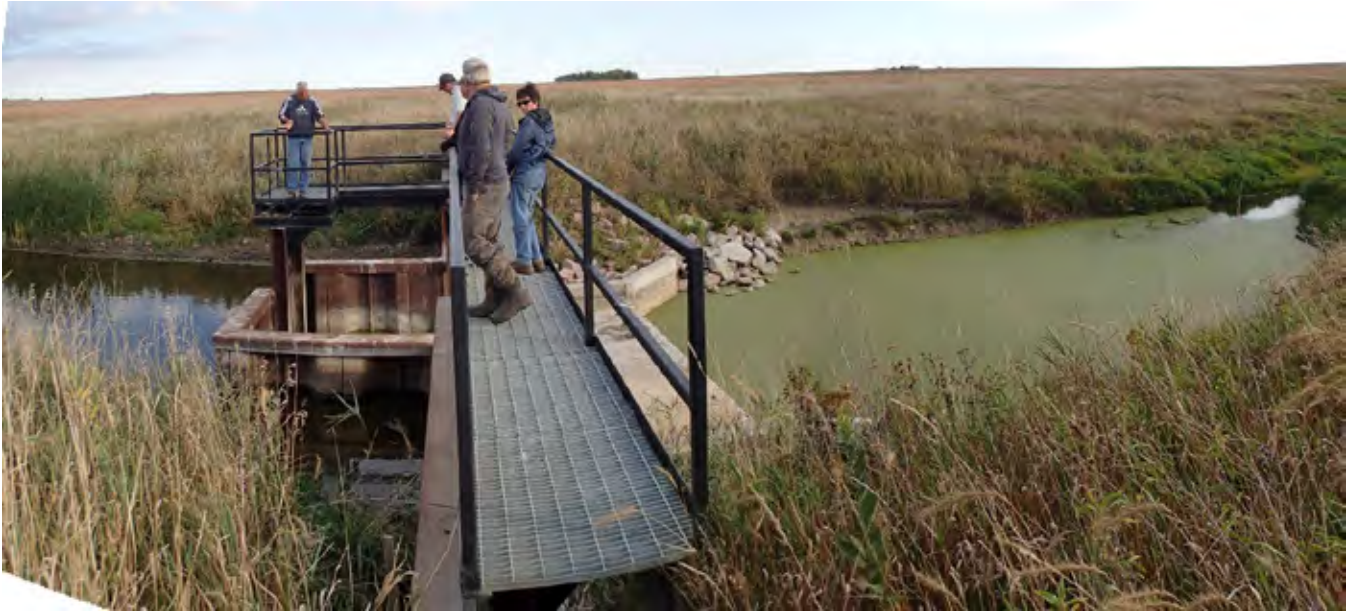
Photo 23-5 Water control structure installed to facilitate water level manipulation in the wetland upstream (left in the photo).
