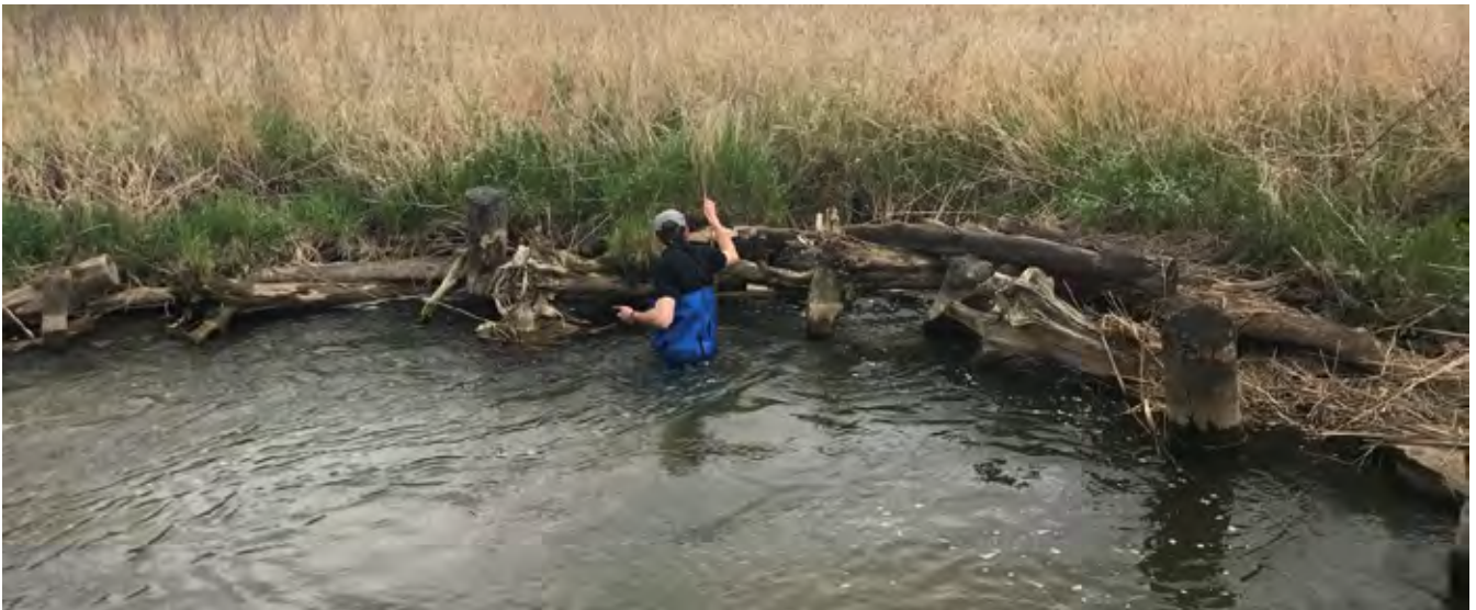
Photo 7-4 5/21/2018 photograph of toewood installation. Large voids present in ~7 year old installation, but bank is stable.
