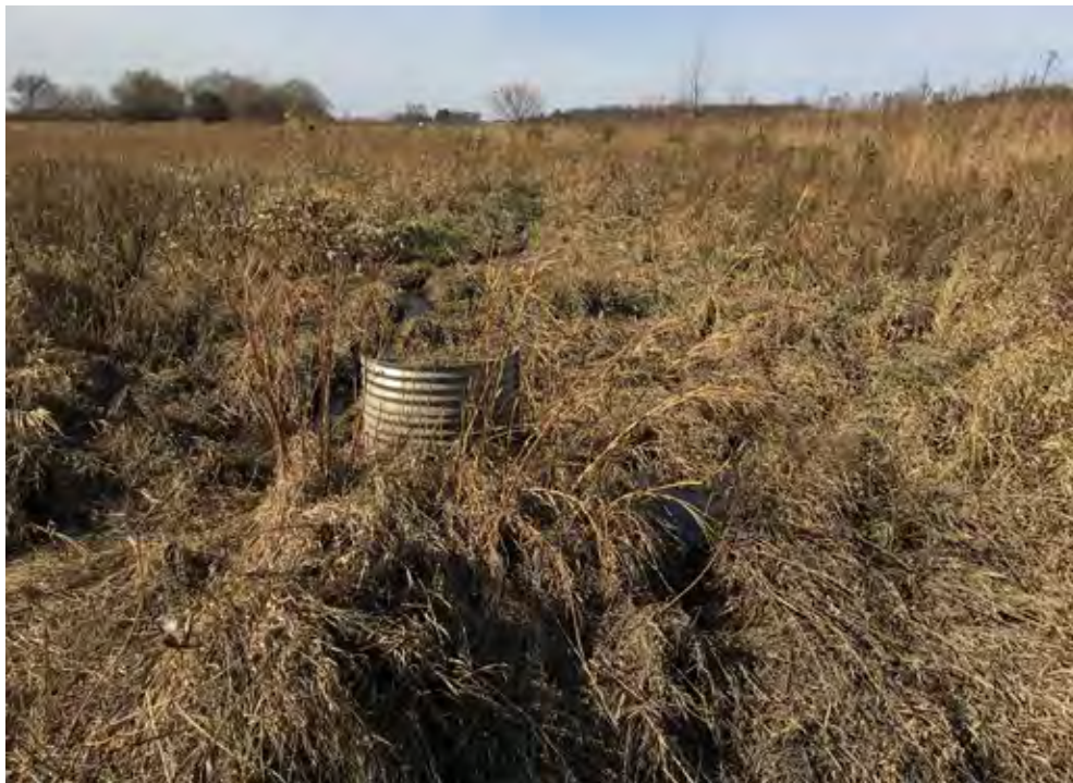
Photo 3-4 Outlet structure of Geomaat retention wetland, 10/24/2018.
