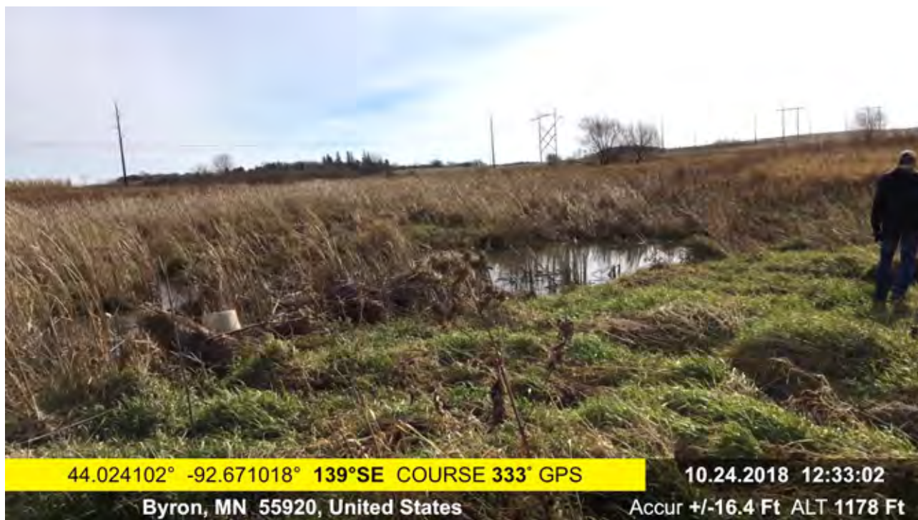
Photo 2-1 Retention basin at inlet, 10/24/18.
