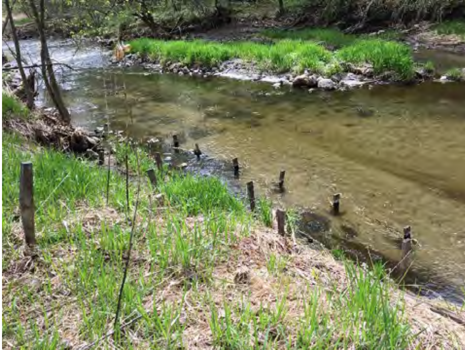
Photo 6-2 Stakes for erosion control blanketing sticking to far out of the ground.
