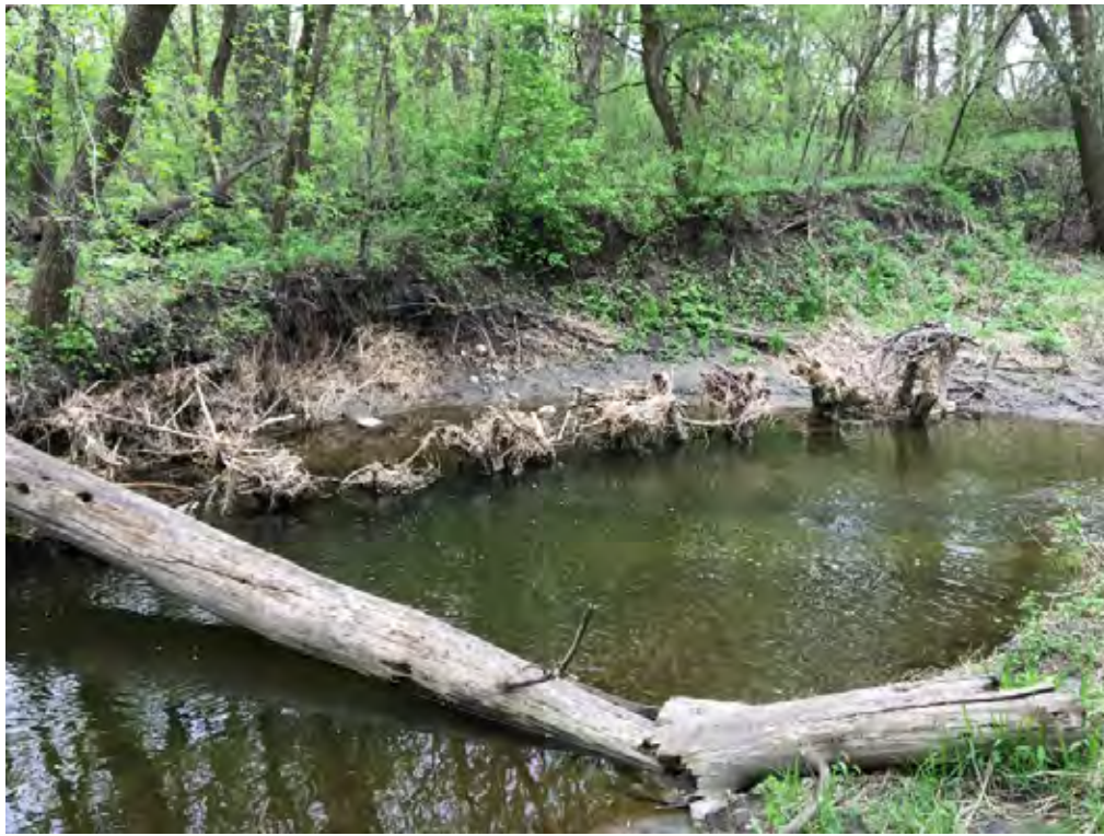
Photo 6-16 Failed tree pin structure. 5/14/18.
