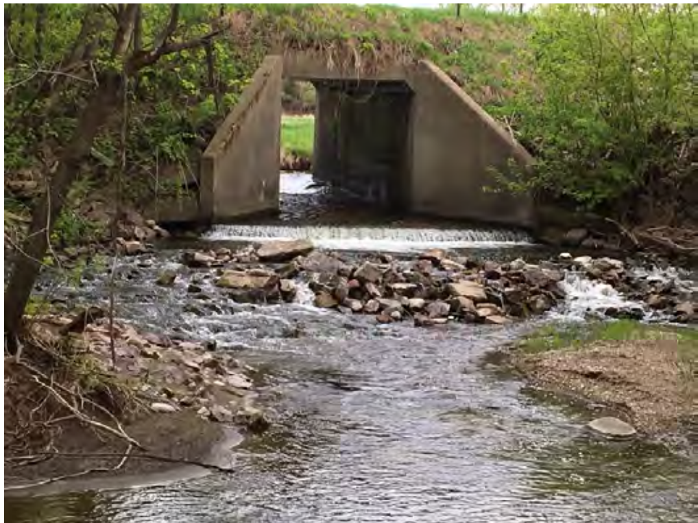
Photo 6-13 Partial failure of fish passage riffle at 280 th Ave culvert, fish passage is still possible. 5/14/18.
