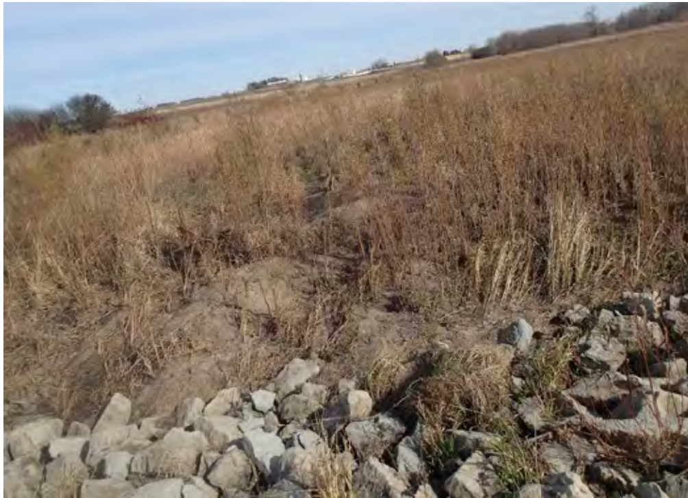
Photo 3-3 Sediment capture observed at bottom of inlet spillway, 10/24/18.
