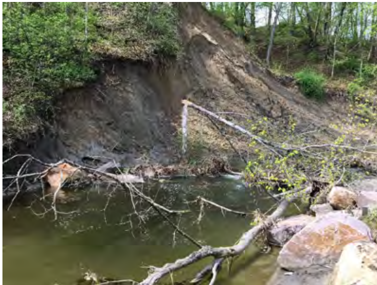
Photo 6-5 Top photo taken 6/6/16 during CPL monitoring site visit, compare to same bank in photo below taken 5/14/18. Significant bank failure and erosion between photos, no structures or stabilizing treatments were applied directly to this bank.
