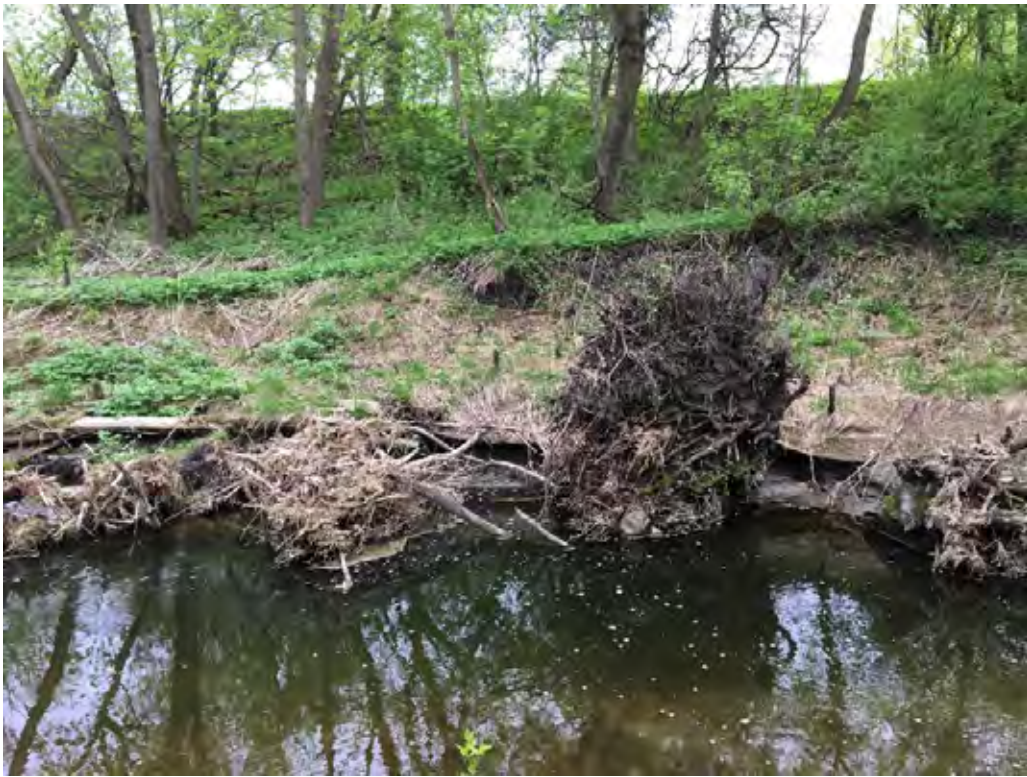
Photo 6-14 Toe wood sticking well out of the water and higher than neighboring pieces possibly causing the erosion in-between the root wads. 5/14/18.
