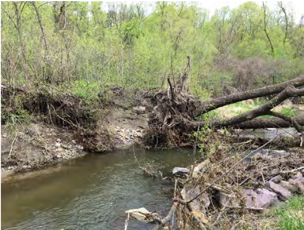
Photo 6-10 Structures at eastern end of project altering stream pattern, pushing flow into banks and causing erosion. 5/14/18.
