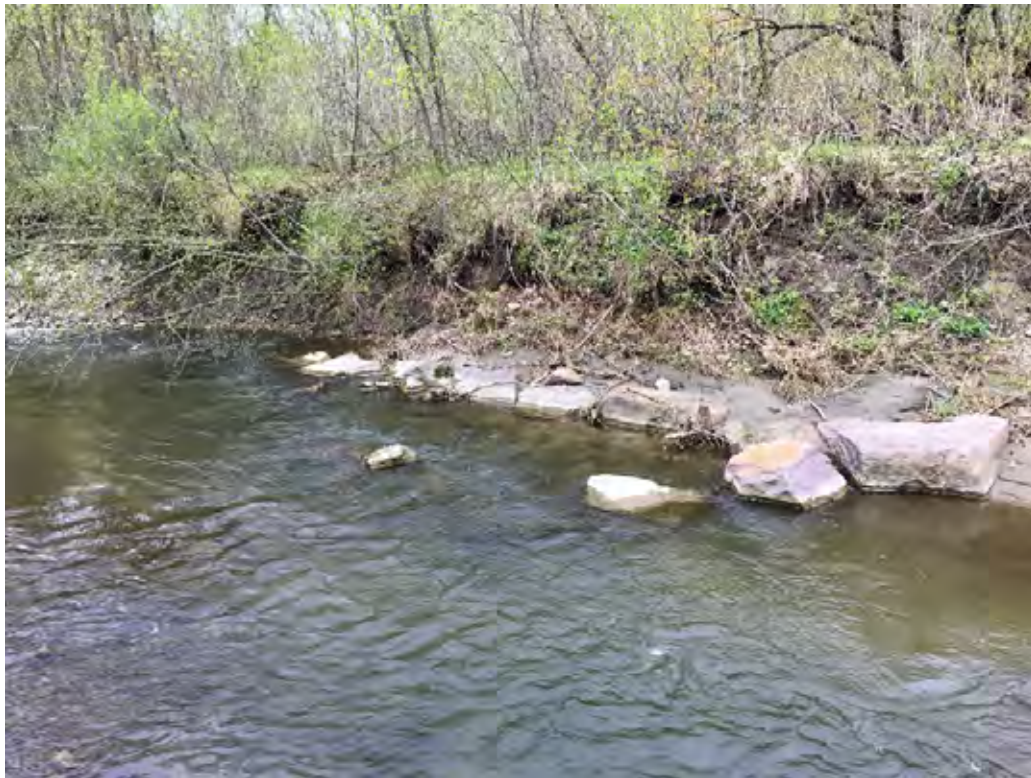
Photo 6-11 Structure at eastern end of project has blown out. 5/14/18.
