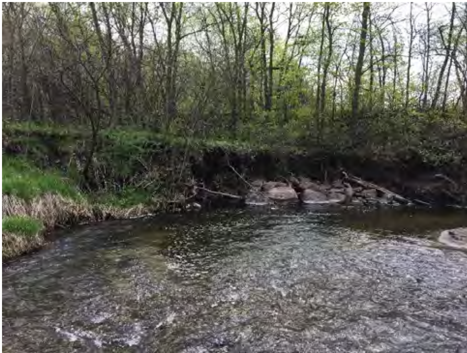
Photo 6-3 Erosion occurring on upstream end of bank stabilizing treatment.
