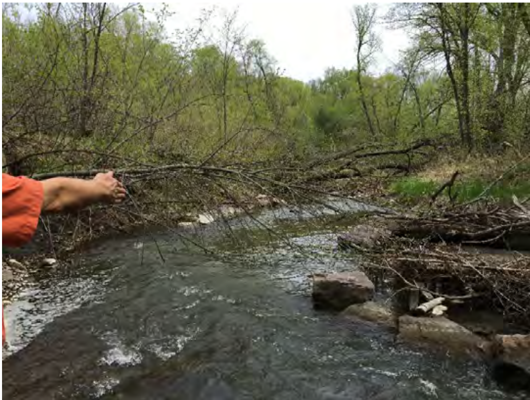
Photo 6-9 Structures at eastern end of project altering stream pattern, pushing flow into banks and causing erosion. 5/14/18.
