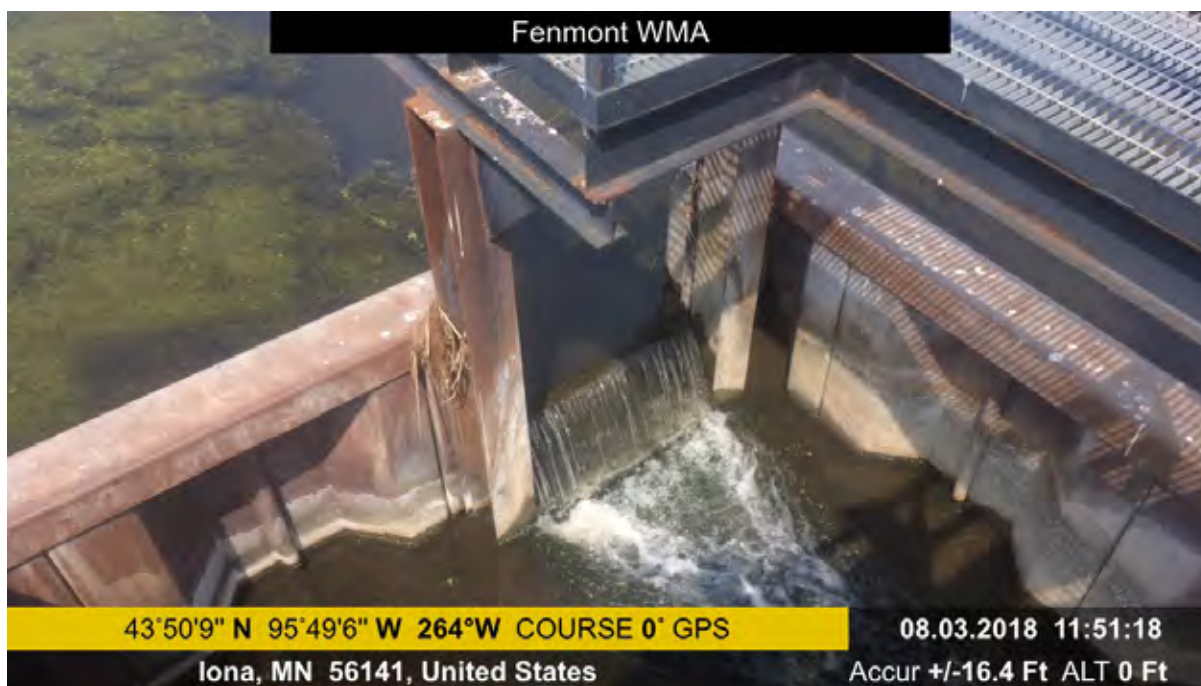
Photo 23-1 View of control structure with sheet piling and stop log structure. Most stoplogs were removed at the time of the field visit to mimic a summer drawdown intended to stimulate vegetation in mud flat conditions.
