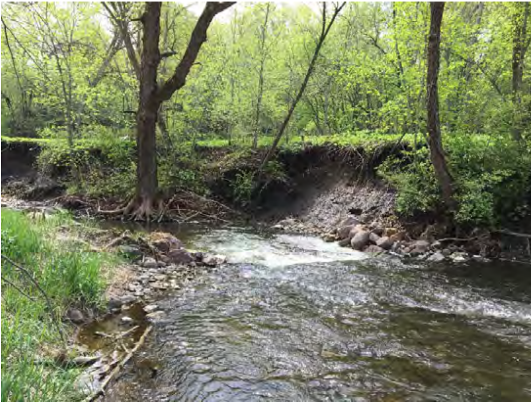
Photo 6-6 Vane creating pool and fish habitat but constructed at wrong angle and directing flow into the bank. 5/14/18.
