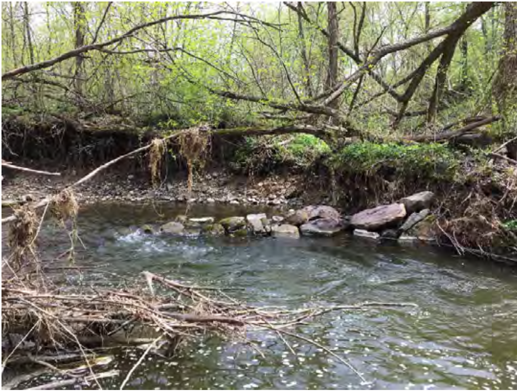
Photo 6-8 Structure diverting flow away from eroding bank. 5/14/18.
