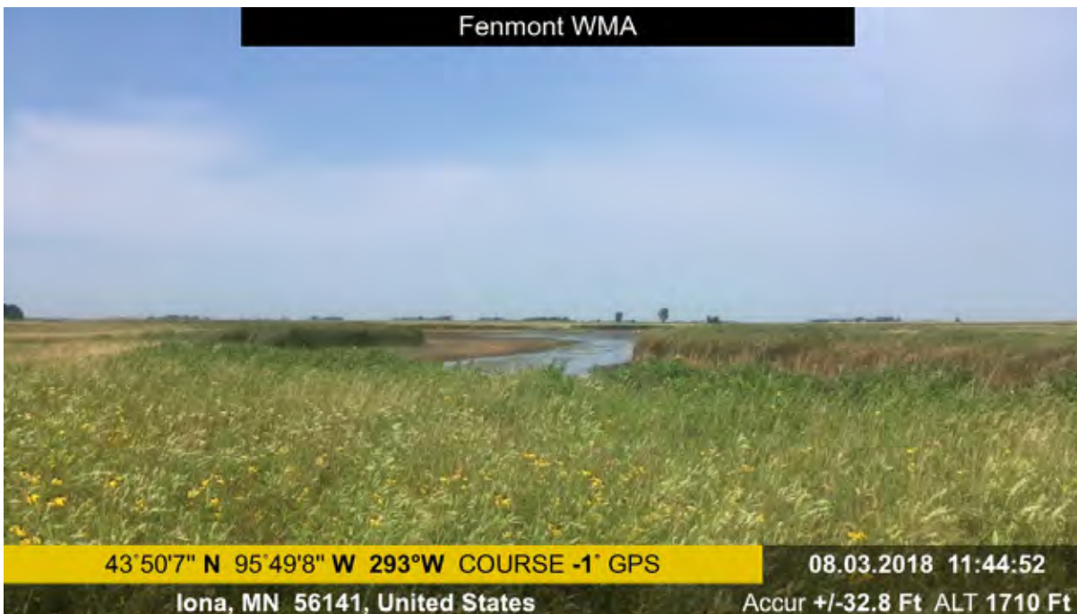
Photo 23-2 View looking northwest from the berm near the wetland outlet structure, showing the wetland during draw down condition.
