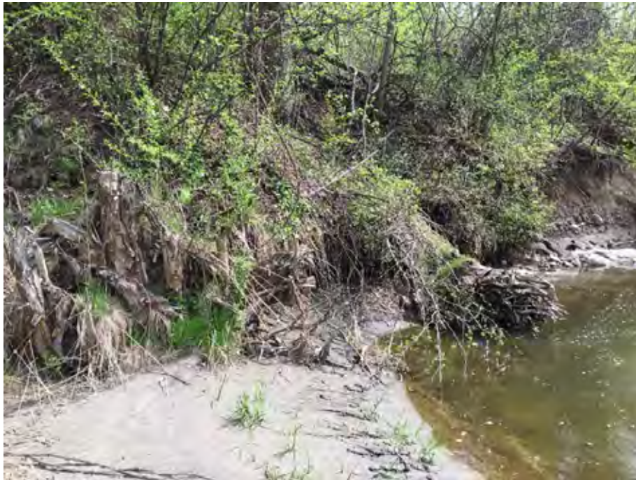
Photo 6-4 Toe wood currently high and dry due to sedimentation from an upstream structure changing the direction of flow.
