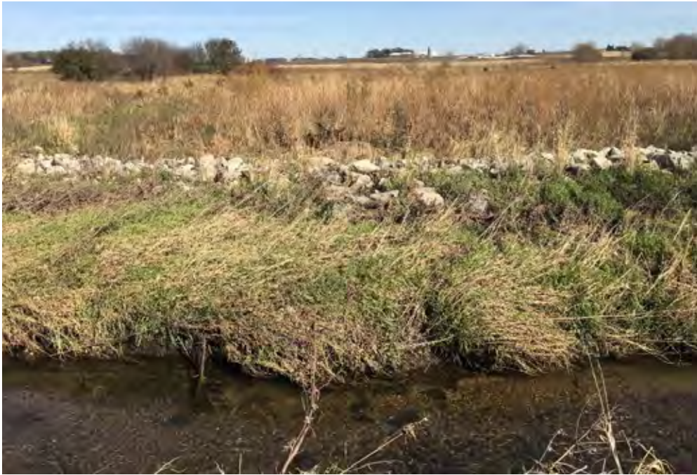
Photo 3-1 Spillway at upstream end of retention basin, 10/24/18.
