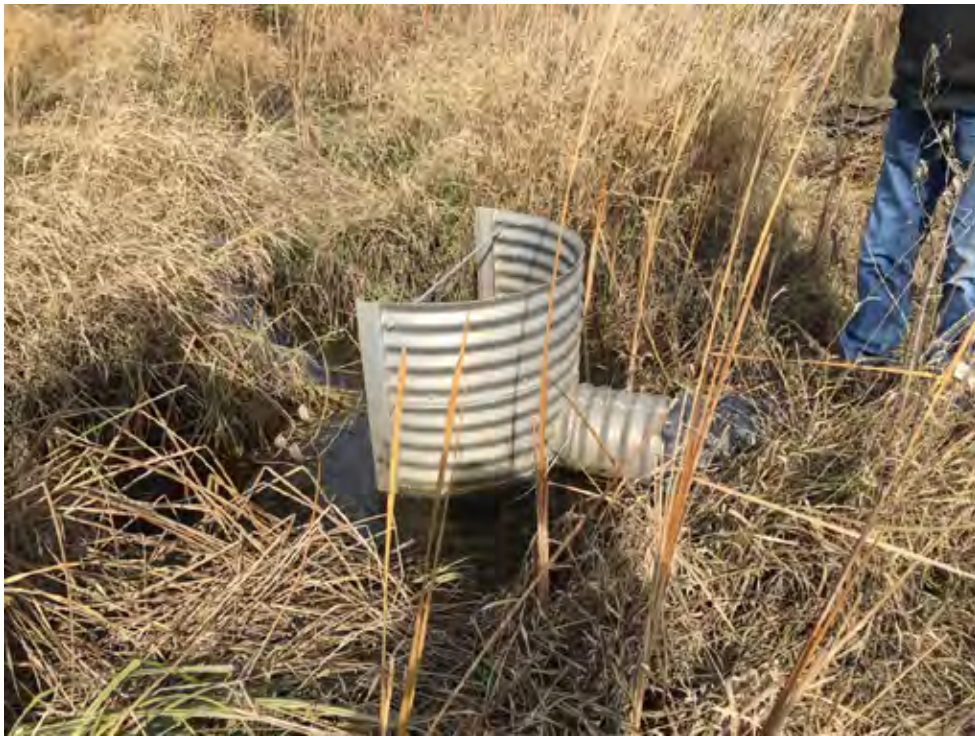
Photo 2-3 Outlet structure of retention wetland.
