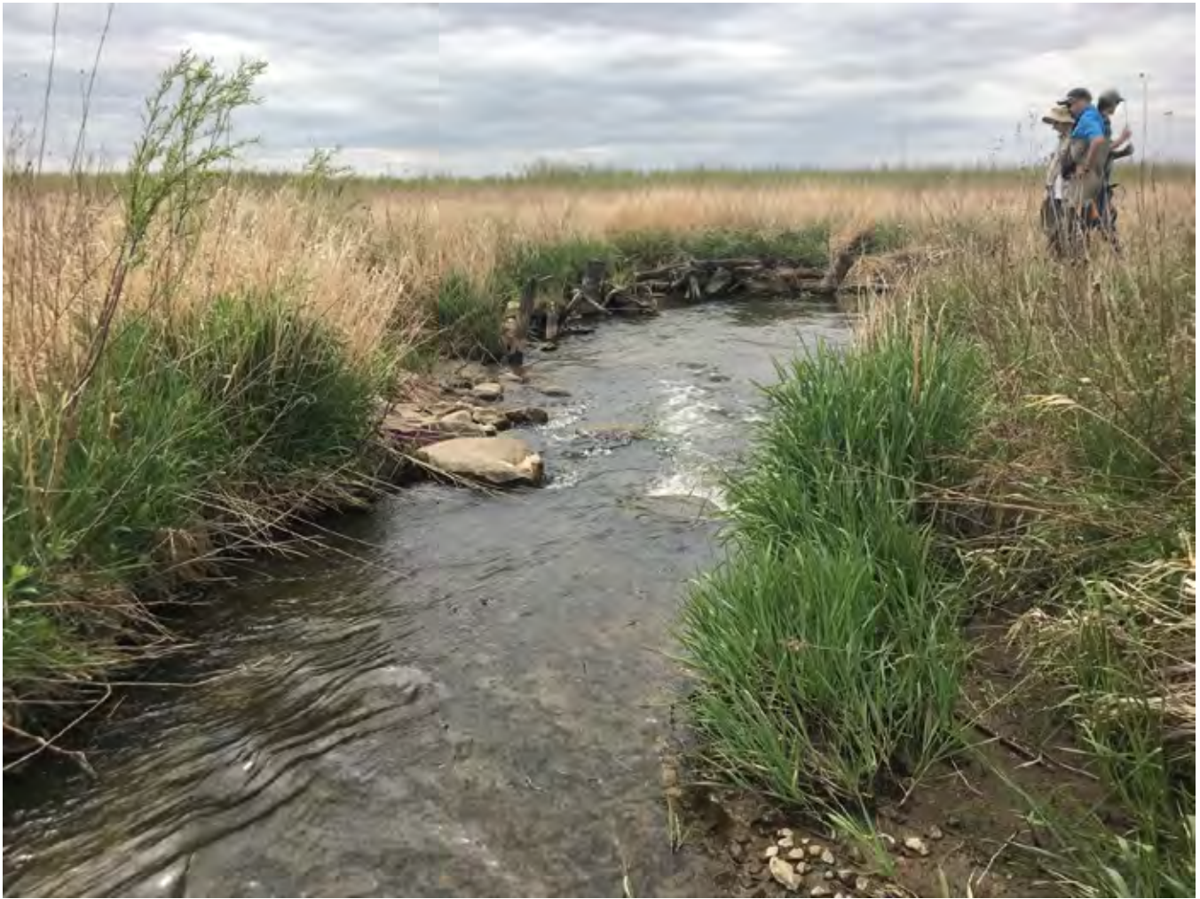
Photo 7-5 5/21/2018 photograph of a created hammerhead pool with a riffle/grade control structure in the foreground (upstream) and toewood installation in the background (downstream).
