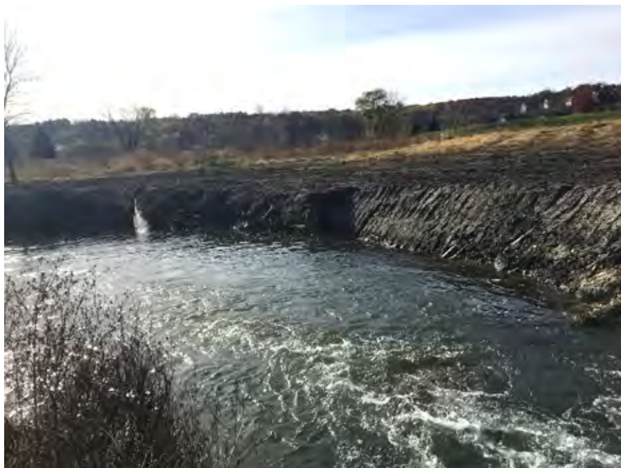
Photo 1-4 View of portion of project reconstruction in 2018.
